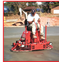
Operator at Work with the Ride-On Trowel
